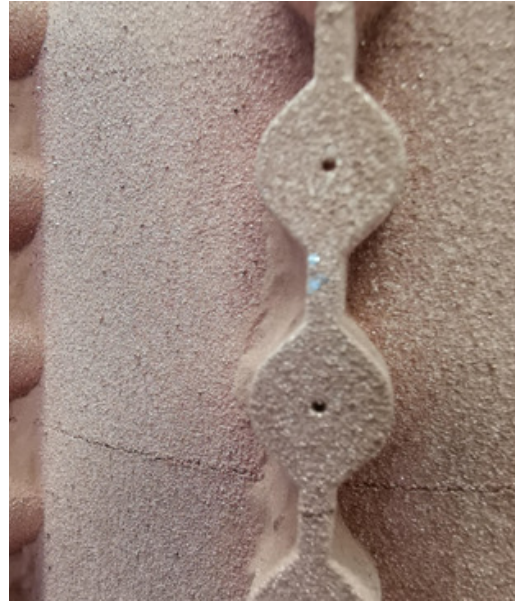
(b) Close-up of cracks
